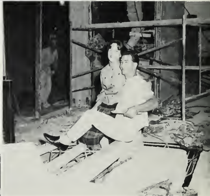
Engravings Editor Pot Welsh and Social Chairman-construction worker Mike Eisenstadt left the office in utter destruction.
